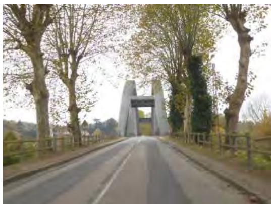
Figure 194 – Pont saint Pierre-du-Vauvray
