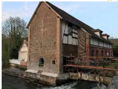
Figure 246 – Moulin à Acquigny (source : CAPLA Architecture)
