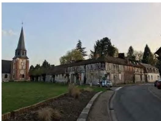
Figure 43 – Site classé d'Acquigny
