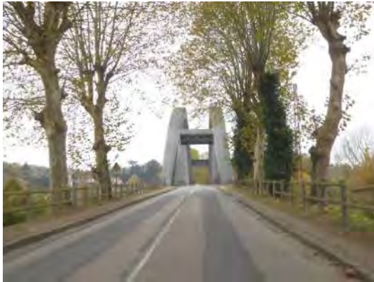
Figure 194 – Pont saint Pierre-du-Vauvray
